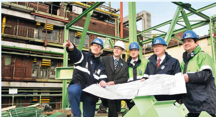
Launch of construction for the world's biggest production facility for carbon nanotubes (CNT) in Leverkusen (from left): Michael Klefisch (Construction Planning), Dr. Ralph Weber (Head of Production), Roland Motzek (Project Manager), Dr. Josef Sanders (Plant Manager) and Dr. Dieter Zeitz (Plant Engineer)
